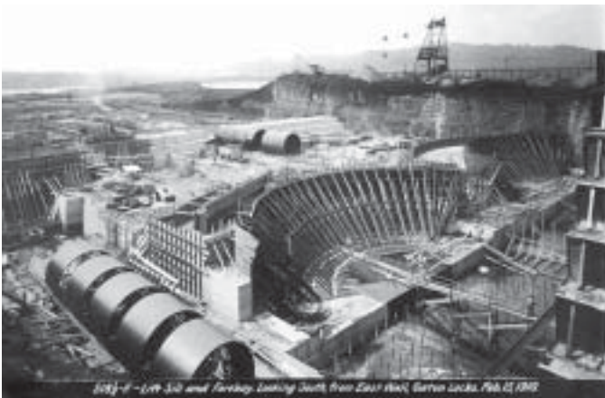
Gatun Locks under construction, Panama, from NICHOLS, A.B. Panama Canal Notebooks, 1882-1920.
