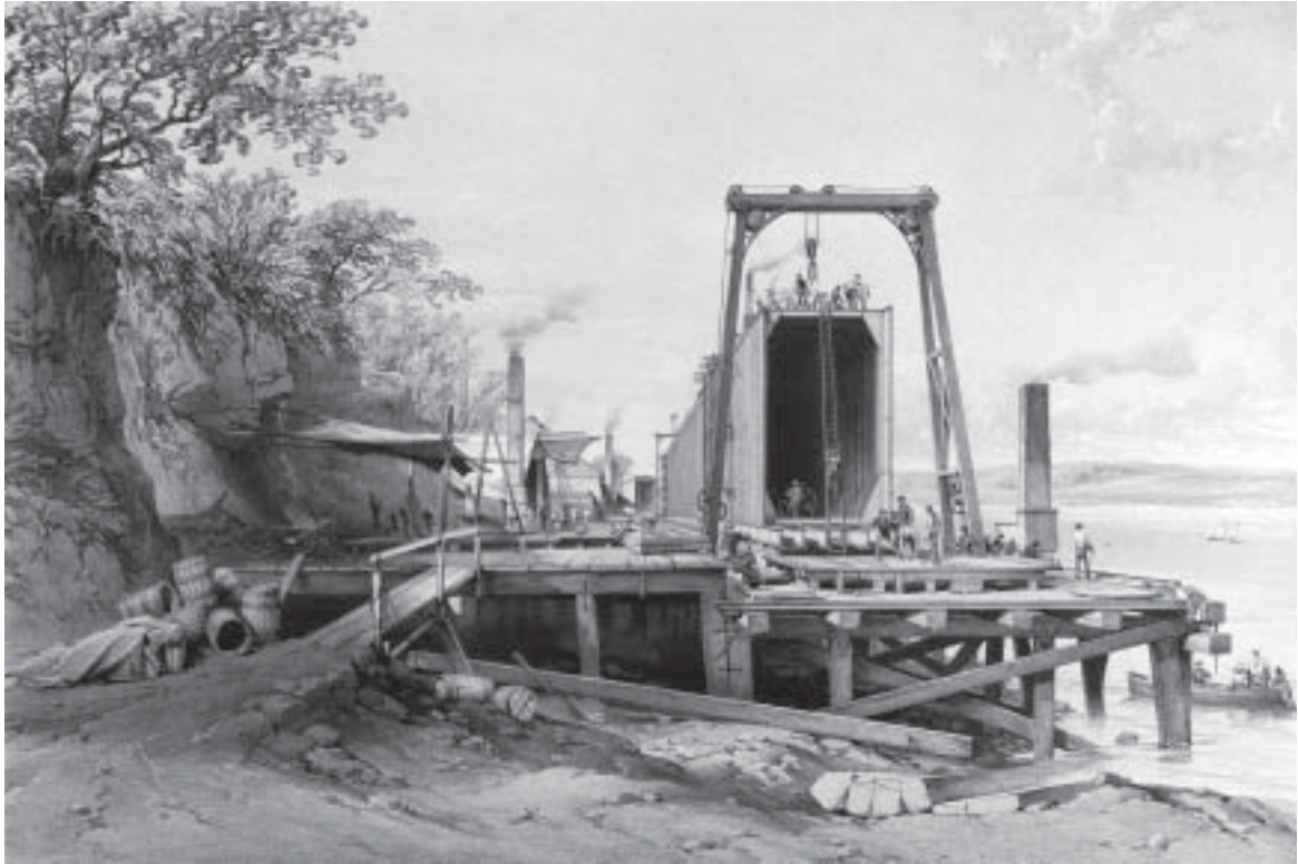
Detail of a tube under construction for the Britannia Bridge, from CLARK, E. The Britannia and Conway Tubular Bridges. London, 1850.
